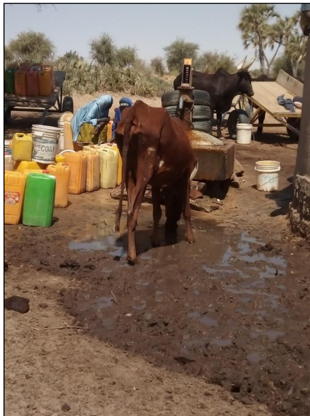
Photo 3: Hand Pump with Poor Drainage – Galmeri Village in Mazamni Commune, Zinder Region
