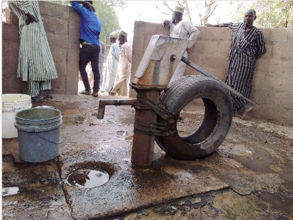
Photo 2: Handpump with Poor Drainage – Makera Village in Gouchi Commune, Zinder Region
