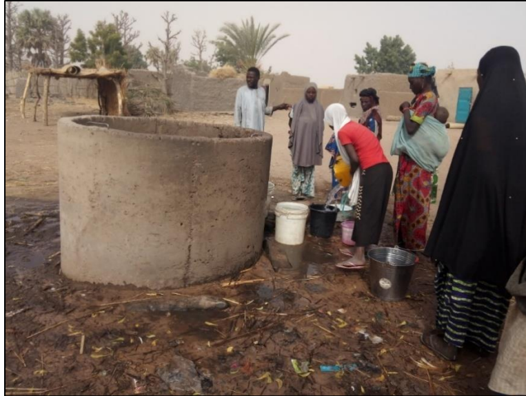
Photo 4: Poor Drainage Around a Hand-Dug Well – Magelwa Kaba Village in Gouchi Commune, Zinder Region
